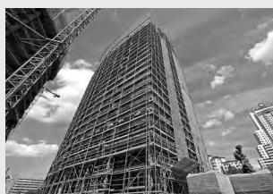
working scaffolds facade
