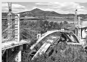
bridge formwork
