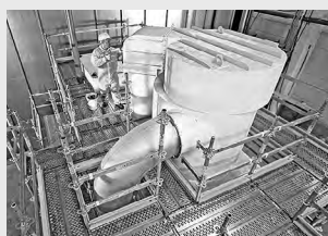
working scaffolds industry
