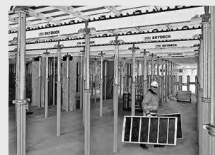
slab formwork
