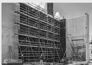
working scaffolds construction
