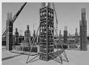
column formwork
