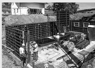
wall formwork
